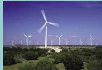
Courtesy of General Electric
